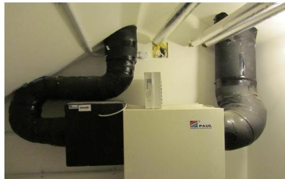
Fig 2. Passivhaus design specifies vapour retardant insulation, to prevent condensation forming inside or outside the ventilation ducts
